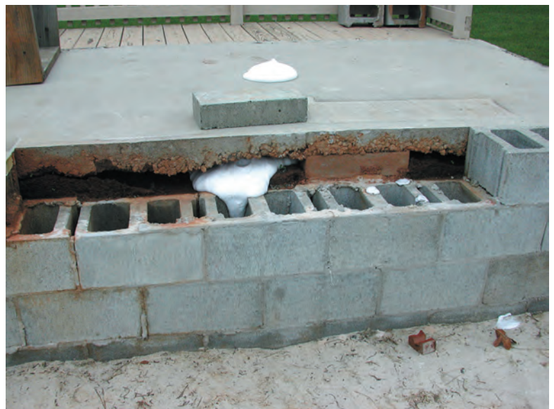
Figure 18. Foaming can be an effective treatment technique when treating areas containing voids, such as those under some porches (shown here) and inside walls, because the foam expands to treat all surfaces.
